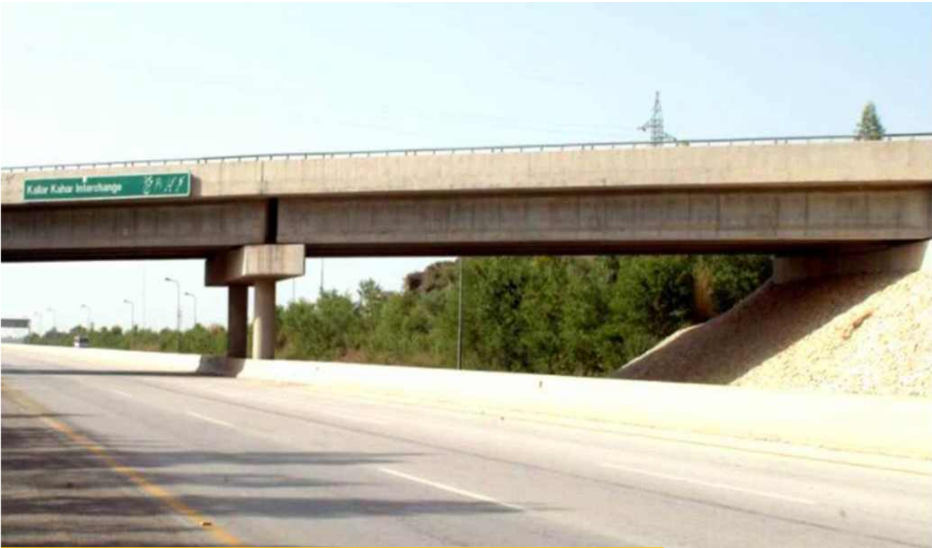
POST TENSIONED BRIDGE – MOTOR WAY PAKISTAN
