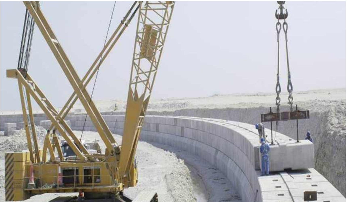
ERECTION OF PRECAST ELEMENTS – LUSAIL DEVELOPMENT PROJECT
