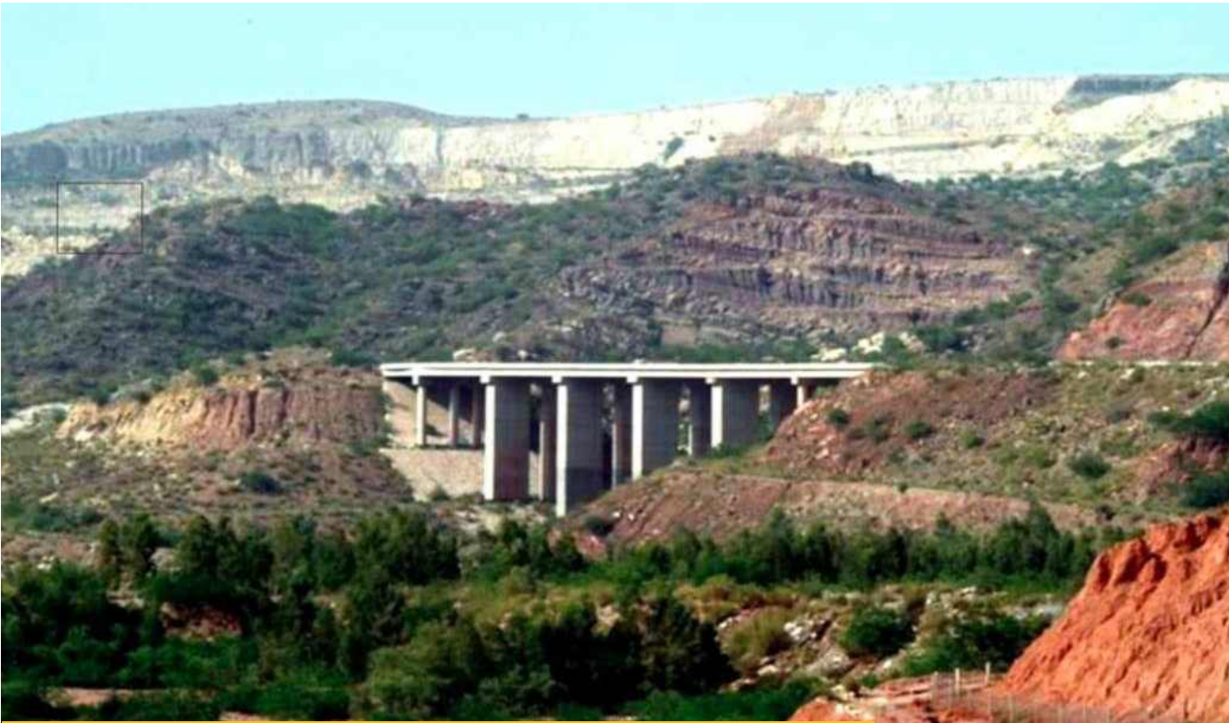
POST TENSIONED BRIDGE – MOTOR WAY PAKISTAN
